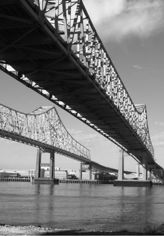
Truss Bridges Terry Poche/Shutterstock
