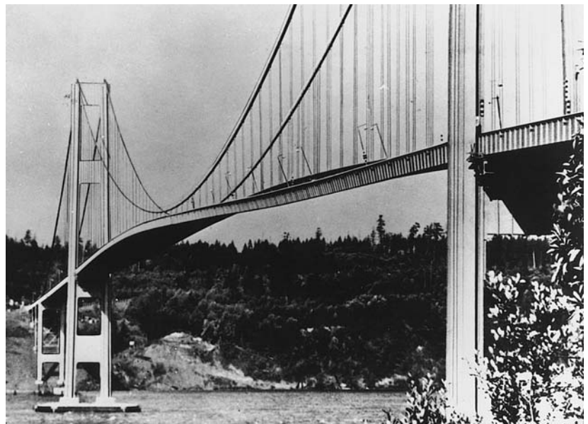
FIG. 1.5 Tacoma Narrows Bridge Oscillating before Its Collapse in 1940 Smithsonian Institution Photo No. 72-787
