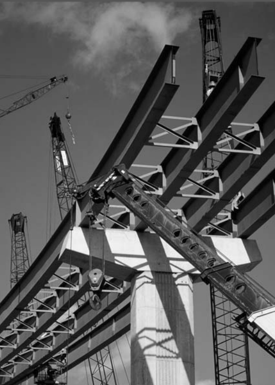
Bridge Construction on an Expressway
