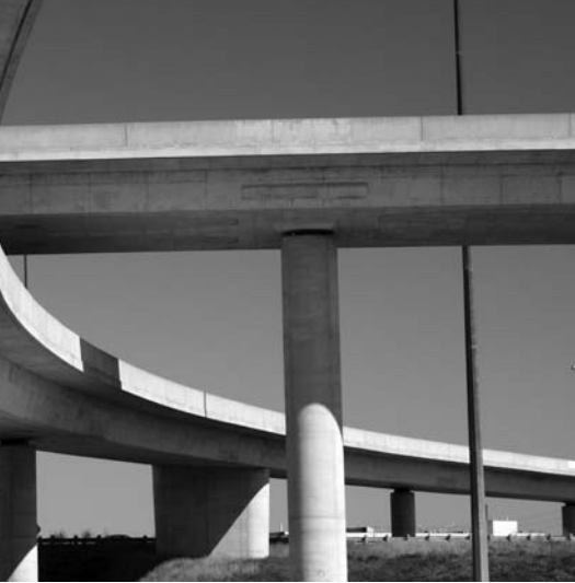
Continuous Beam Bridges
