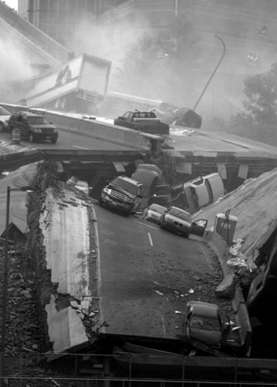
Interstate 35W Bridge Collapse in Minnesota (2007)
